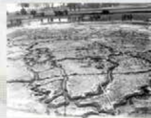
Scale reproduction of the trenches at Vimy Ridge.
